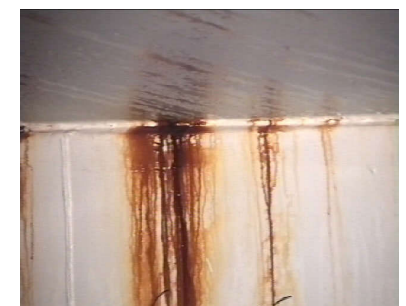
Seam Corroded
